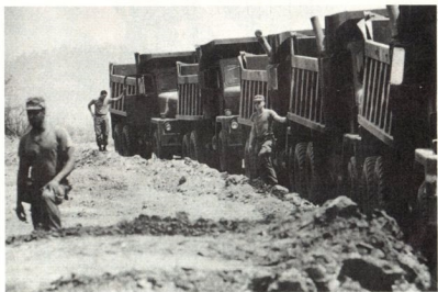
U.S. airfield being built in Jamastran, Honduras, 20 miles from Nicaragua
